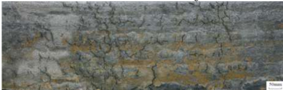
Fig1. The macroscopic feature of surface cracks.
