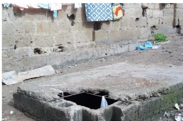
Plate 4.9: Showing dilapidated Septic Tank in the study area. Source: Author's Field Survey, 2018
