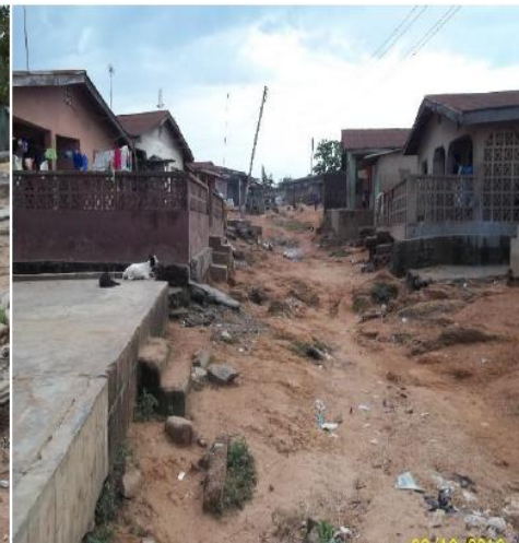
Plate 4.15: Access road in the study area
