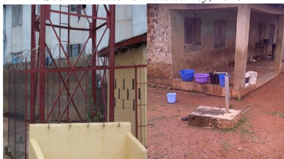
Plate 4.6: Showing a nonfunctional borehole in the study area.
