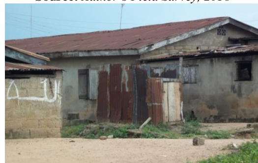
Plate 4.3: Showing external toilet and bathroom Source: Author's Field Survey, 2018
