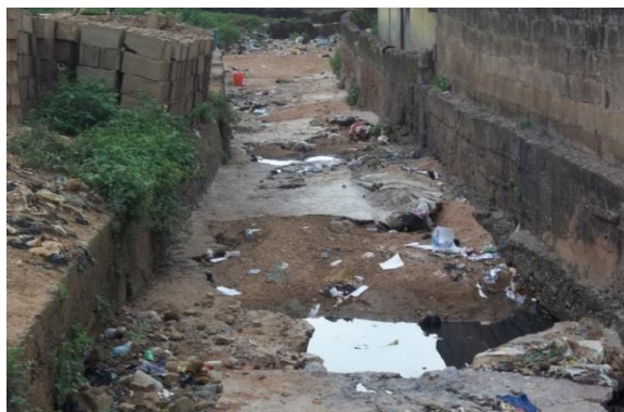
Plate 4.8: Showing Dilapidated drainage System Source: Author's Field Survey, 2018
