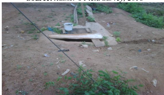
Plate 4.7: Showing an unprotected hand dug well in the study area.
