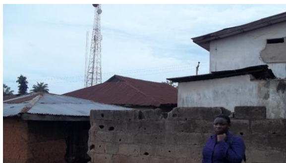
Plate 4.2. Showing roofing material used in the study area
