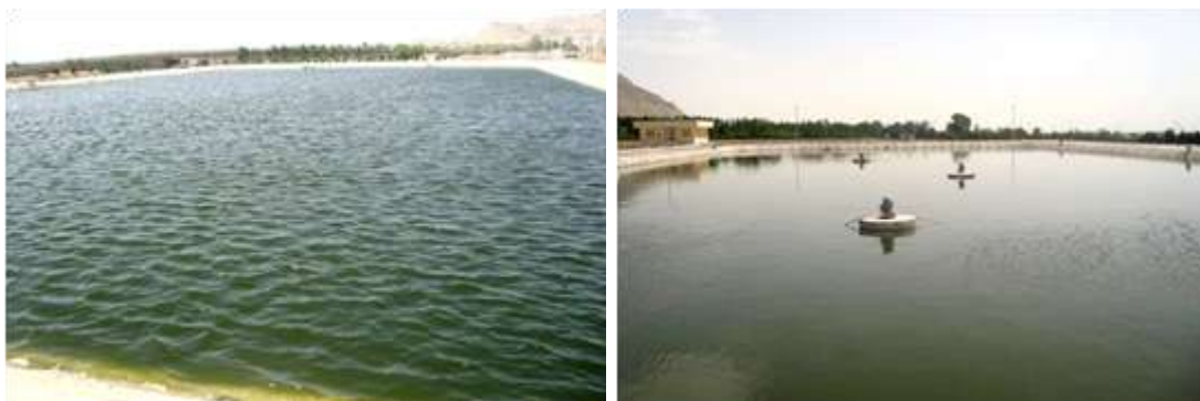
Figure1. Exhaust from collecting and treatment pools of wastewater from Isfahan University of Technology
