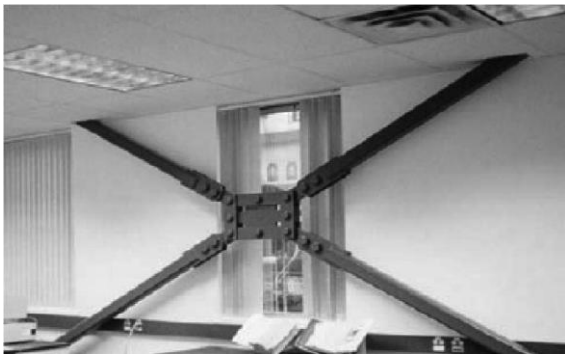
Figure1. Friction damper in a steel building
